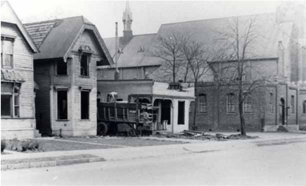
1939: Demolition of neighborhood houses to make room for the Third Order Hall
